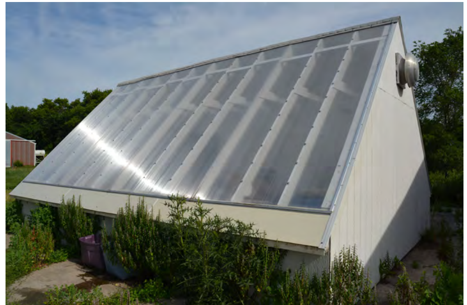
Full-height 12' polycarbonate panels attached to wood frame at Lorri Maus' greenhouse Photo: Jody Rader
