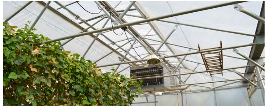
Double 6mil polyethylene glazing at Whitewater Gardens Photo: Jody Rader
