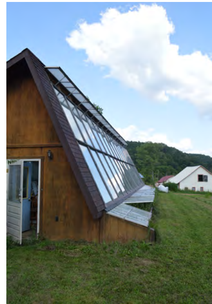
Ridge ventilation at Sweet Earth Farm Photo: Jody Rader
