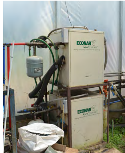
Geothermal Heating System at Whitewater Gardens Photo: Jody Rader
