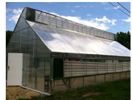
Poly-Vent sidewall ventilation/insulation at Lanesboro High School Photo: Jody Rader
