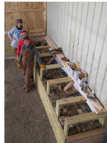
Thermal mass integrated into storage at Paradox Farm (in construction) Photo: Sue Wika
