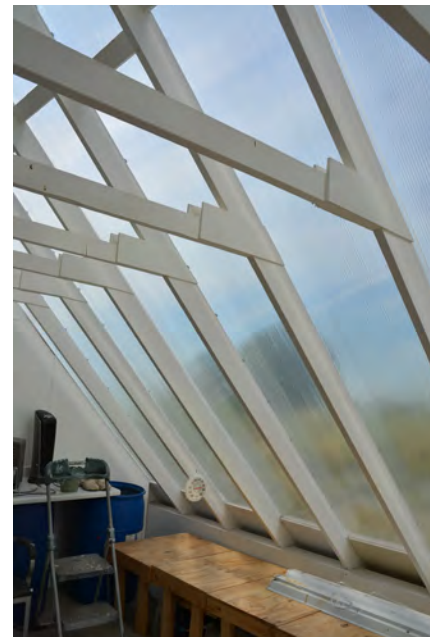
(left) Painted wood frame structure with site-built trusses at Lorri Maus' greenhouse Photo: Jody Rader
