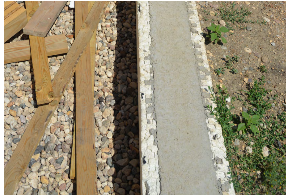
Insulated Concrete Form foundation at Lac Qui Parle Valley H.S. greenhouse. Note EPS insulation on both interior and exterior sides of concrete stemwall. Photo: Jody Rader
