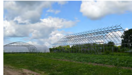
(above) Aluminum frame quonset-style frame for high tunnels at Whitewater Gardens Photo: Jody Rader
